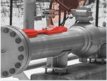
Once a passage has been detected, the LED array will light up. Here, the TRAXALL 620 indicates a pig configured with a 27.3 Hz transmitter has arrived.
